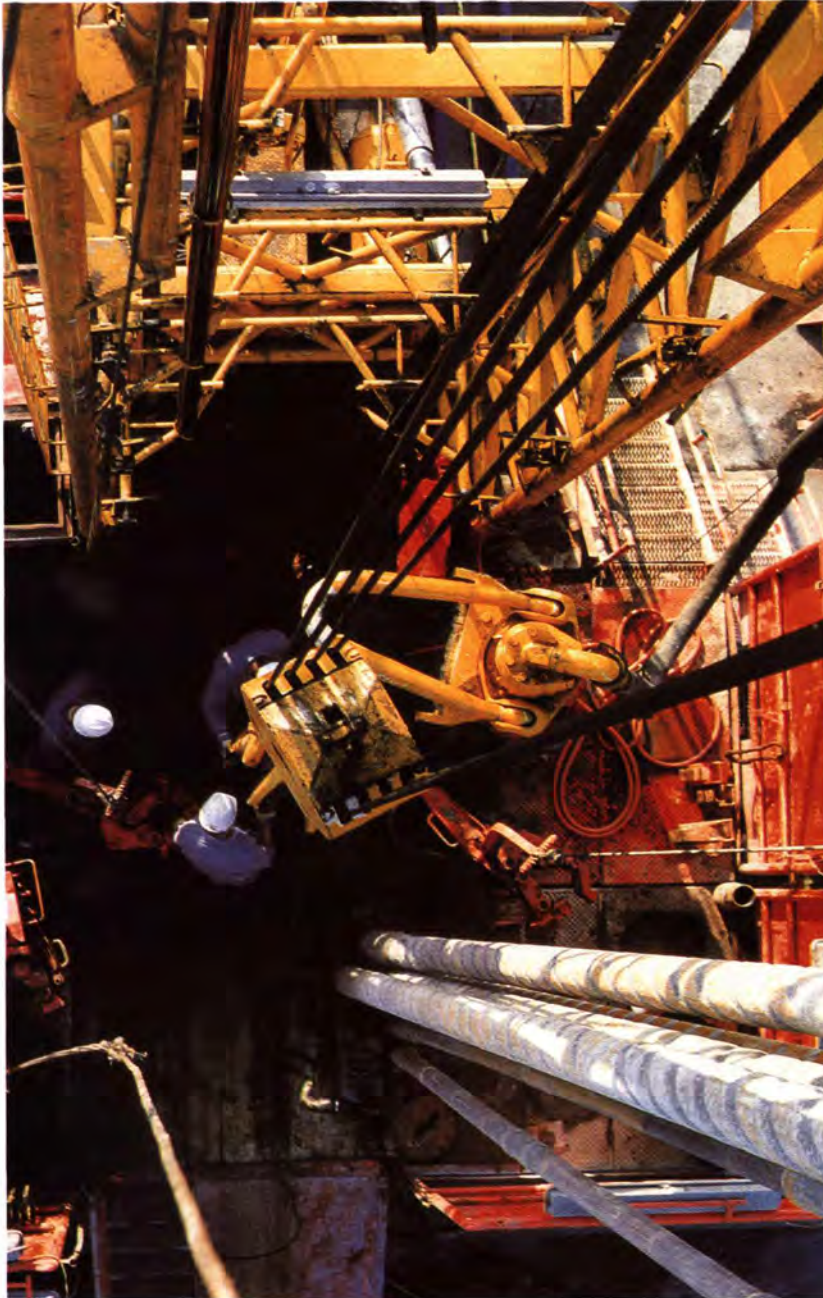
Test drilling at our Adolf van Nassau salt concession near Veendam, the Netherlands, which showed the suitability of salt caverns for gas storage.
